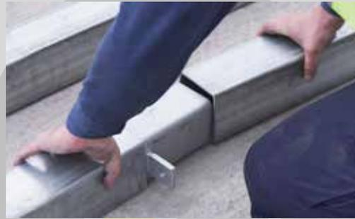
Each arch has a number of sections which are joined using tee joiners. These joiners are designed to be a tight fit and may require force to ensure they are properly located.
