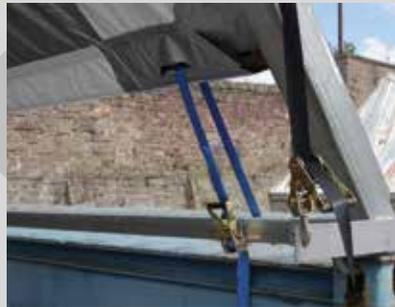
Bring all the ropes together at the far side of the right-hand container and attach to a forklift or similar machine that can pull the cover over. Please note that, whilst this process can be done manually, the tension on the cover must be maintained at all times, especially when it is windy.
