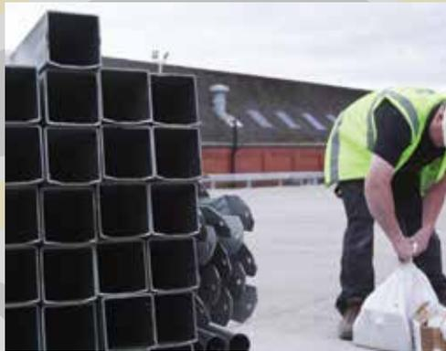
Using the checklist provided in the document pack, carefully check off every component in turn, and place neatly so that each part can be easily identified. This will save a considerable amount of time as the project progresses.
