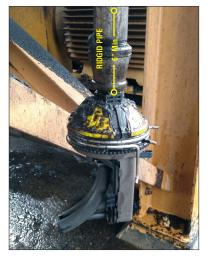
The R75M Debris Sweeping Sprinkler requires a ridgid inlet pipe, at least 6" long.
