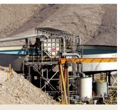
EQUIPMENT EXAMPLE: A clarifier thickener tank can become corroded, reducing mill water availability. Leaks can cause hazardous and costly environment spills that result in fines and employee safety issues.
