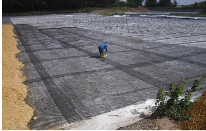
Figure 4. Geogrid T-shape installation
