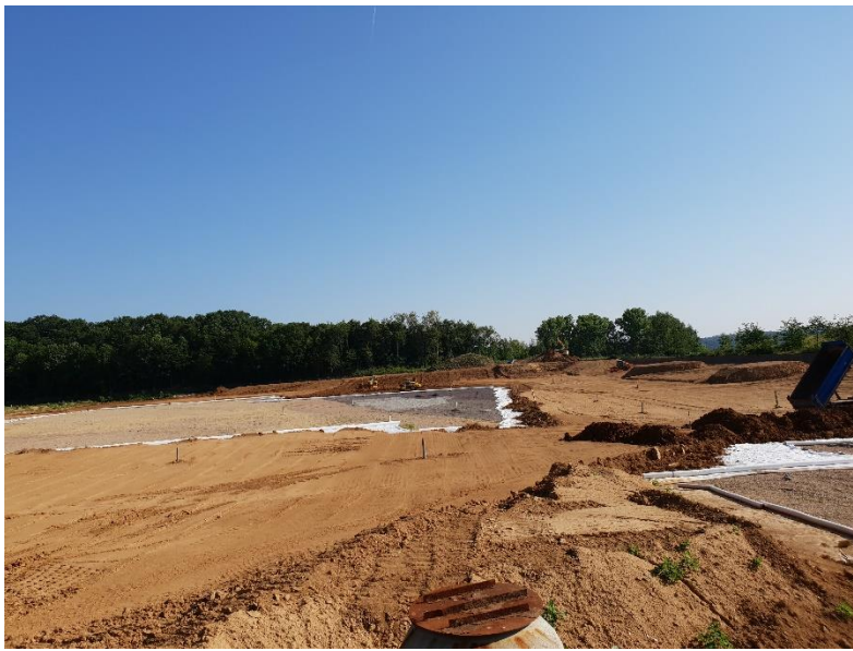
Figure 6. Installation of the top soil
