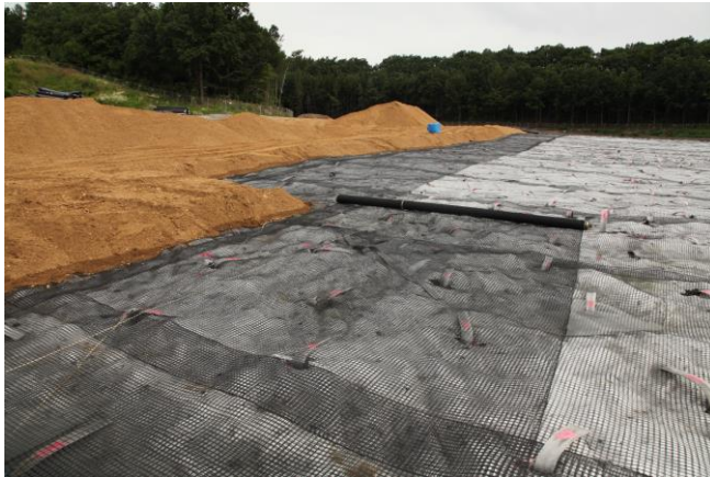
Figure 5. a) Installation of the cover system in the middle region: strip drain installed between the geogrid layers; b) Zoom on the strip drain area after installation
