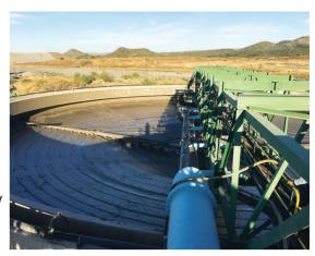
The customer's thickener was constructed in 2011 with the tank manufactured from concrete. The design was that of a centre column with a half span bridge. The bridge was supported on one end at the edge of the thickener, the other on the centre column in the middle of the thickener tank.
