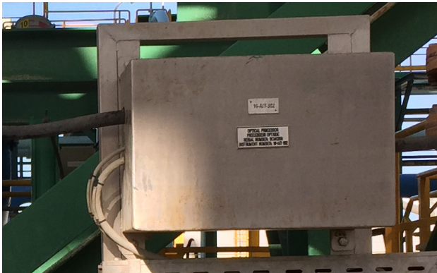
Blue Cube optical processor temperature cover
