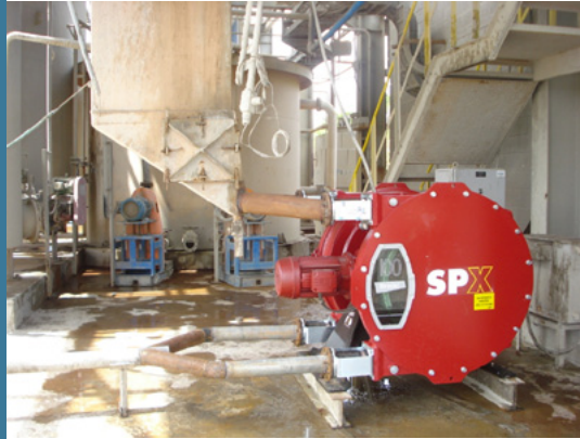
Brexel SPX2100 handles paste backfill @74% solids and 4% cement at Turmalina Mine, Brazil.
